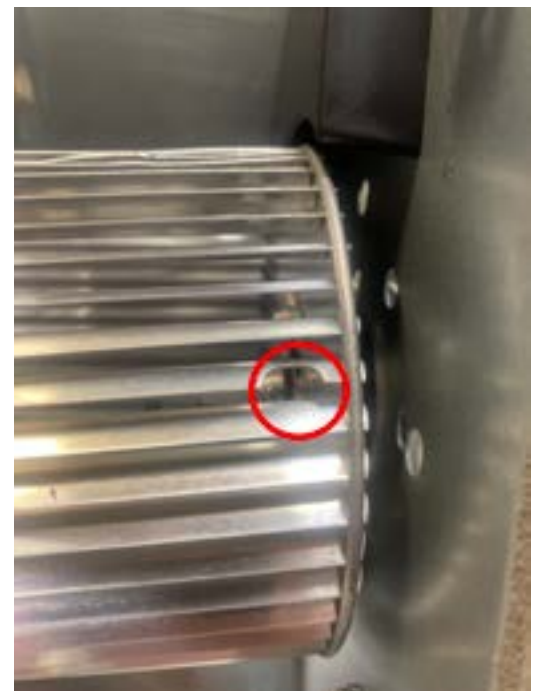
Figure 712 (Loosen Set Screw)
