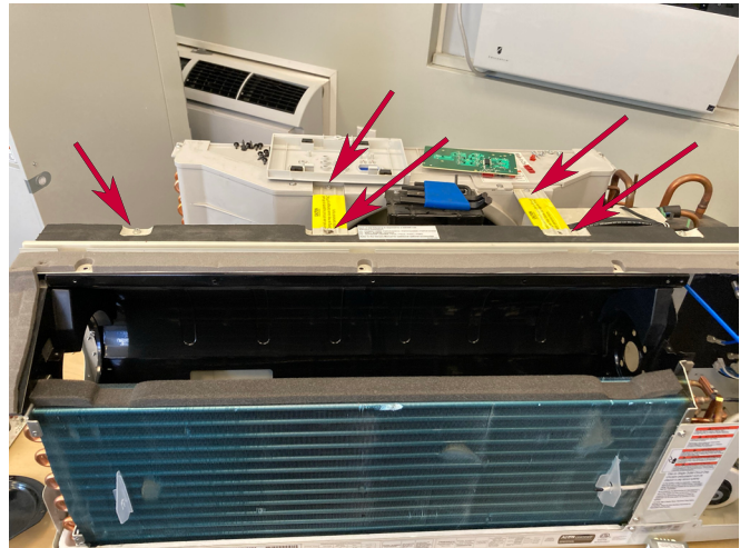
Figure 523 (Remove Top Support Bracket)
