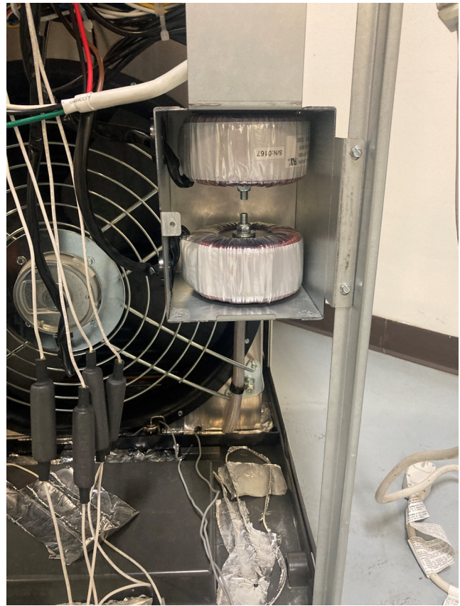
Figure 630 (REPLACE 24,000 BTU TRANSFORMER)
