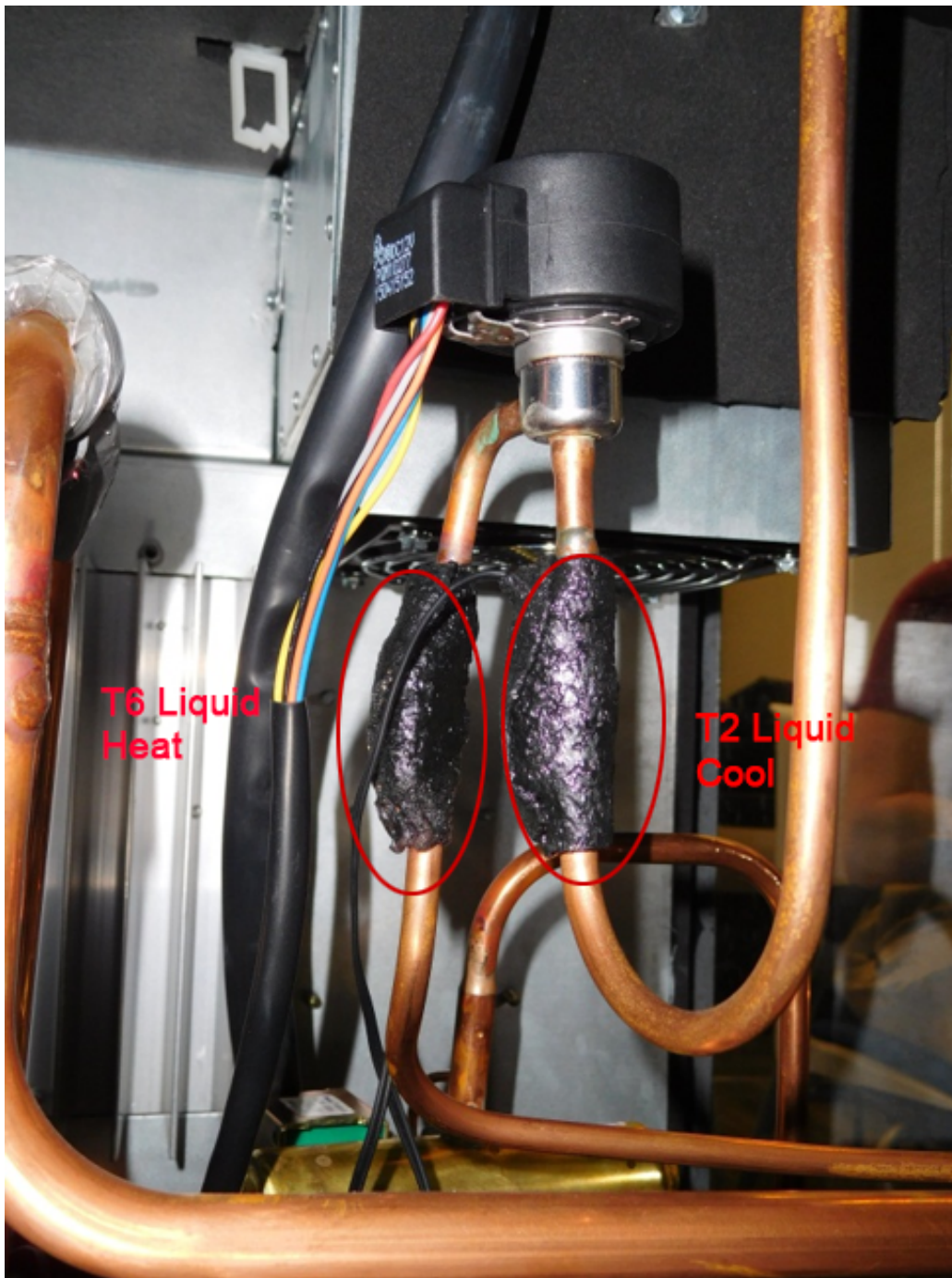
Figure 623 (Thermistor Locations)
